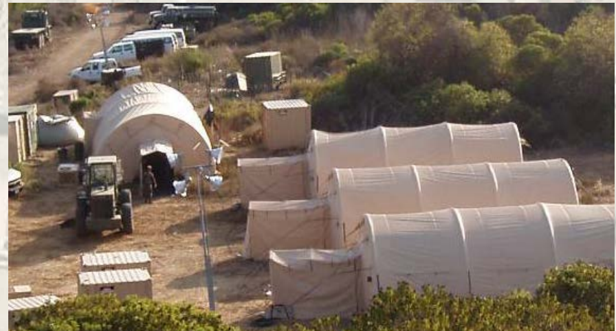
Airbeam Supported Force Provider 150 Soldier Forward Operating Base
